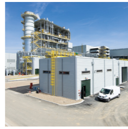
Combined Cycle Power Plant Bayet, France 2008-2010
