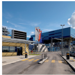
Combined Cycle Power Plant Sparanise, Italy 2005
