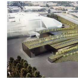
WTE Plant Extension Brescia, Italy 2018-Under Construction
