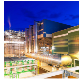
Combined Cycle Power Plant Rizziconi, Italy 2006
