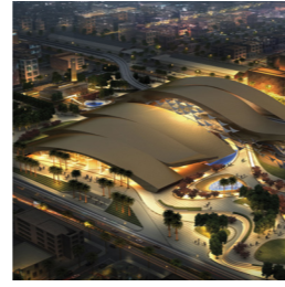
Western Station Riyadh, Saudi Arabia 2013-Under Construction
