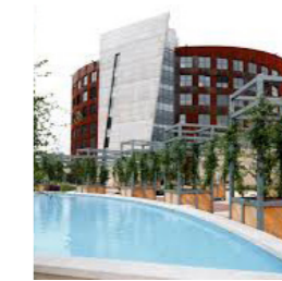
Multy-storey Underground Parking Brescia, Italy 2007
