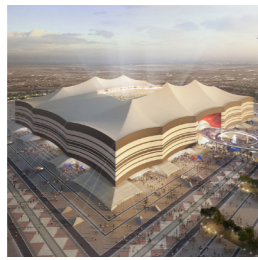
Al Bayt Stadium Doha, Qatar 2015-Under Construction
